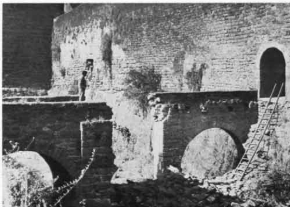
A. Diu: fort, before repairs to culvert. See p. 184
