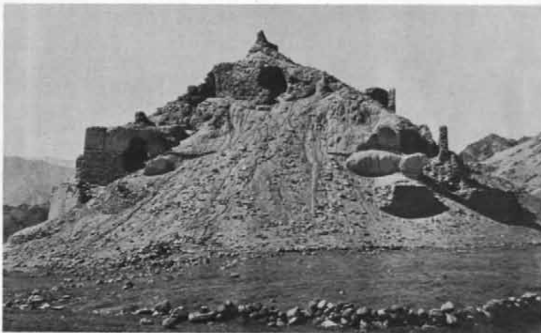
A. Tiserru: stupa, before removal of debris. See p. 182
