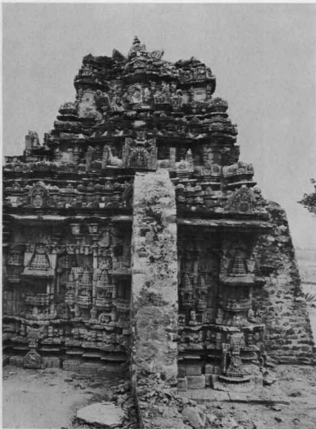
Hirehadagali: Kalleshwara temple, before conservation. See p. 156
