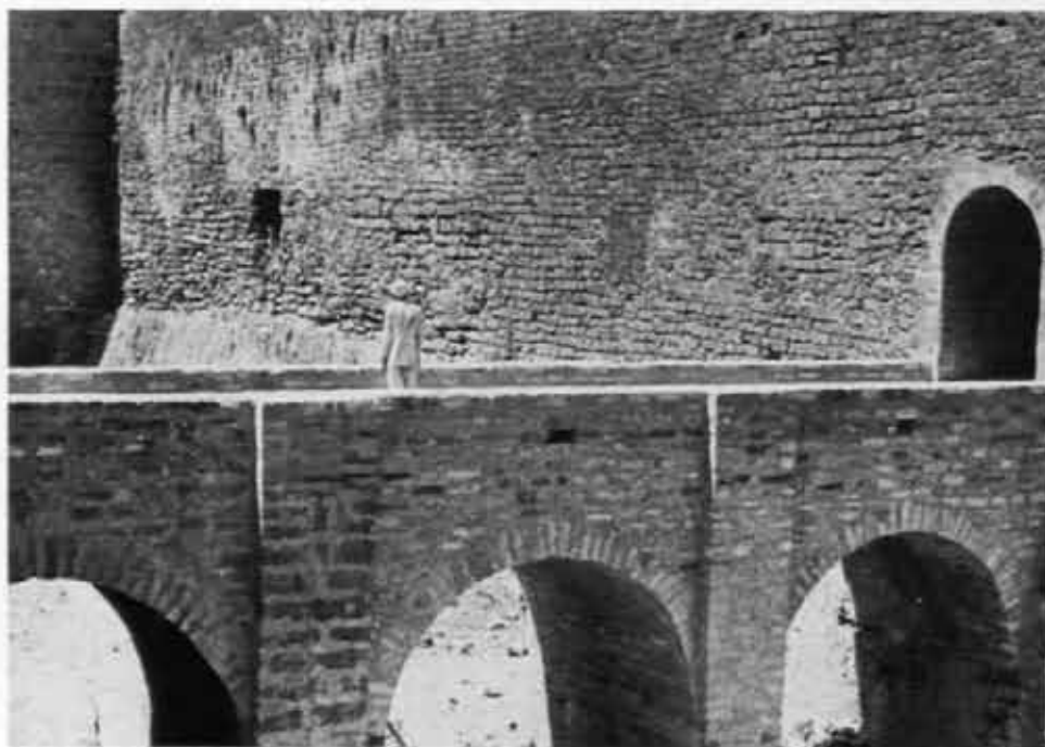
B. Diu: fort, after repair to culvert. See p. 184
