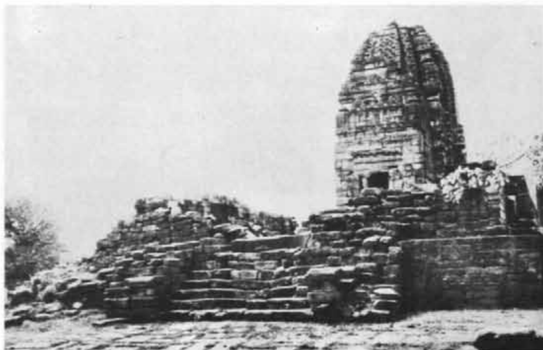
A. Kiramchi: Temple 1, before repairs to entrance. See p. 183
