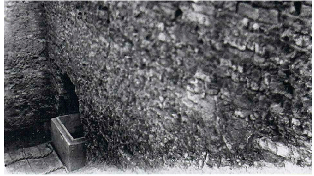
Fig. 12. The coffer in its original position, with enclosing brickwork removed, uncovered, on pull-board.
